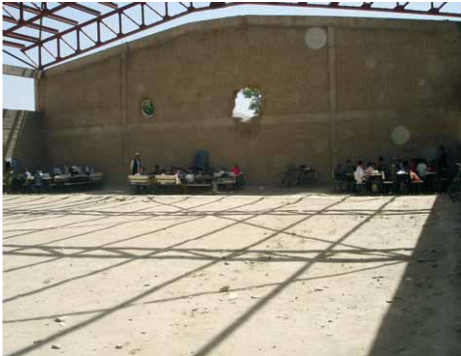
Three classrooms in a storehouse of Qalai Waheed Secondary School
